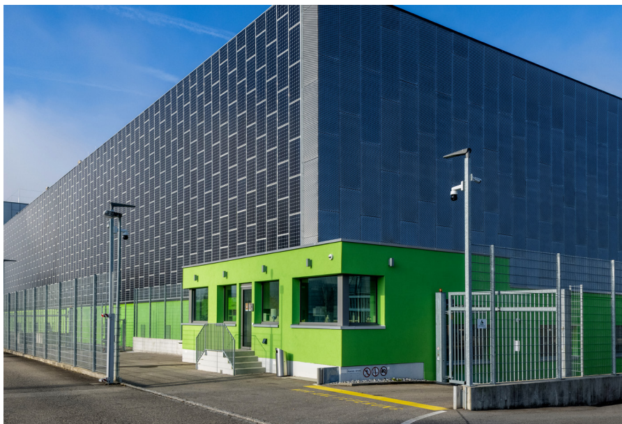
Green Data Centres prioritise sustainability by investing in free cooling and harnessing wasted heat.
